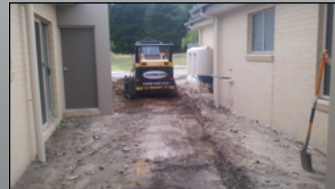
Commercial Earthworks - major or minor
